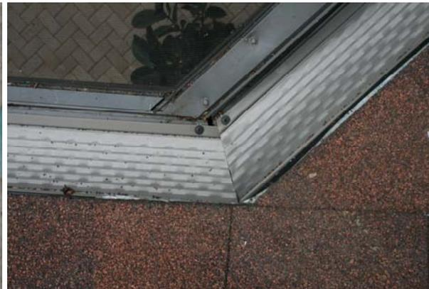
**Panels may be easily cut-to-fit using sheet metal snips**
